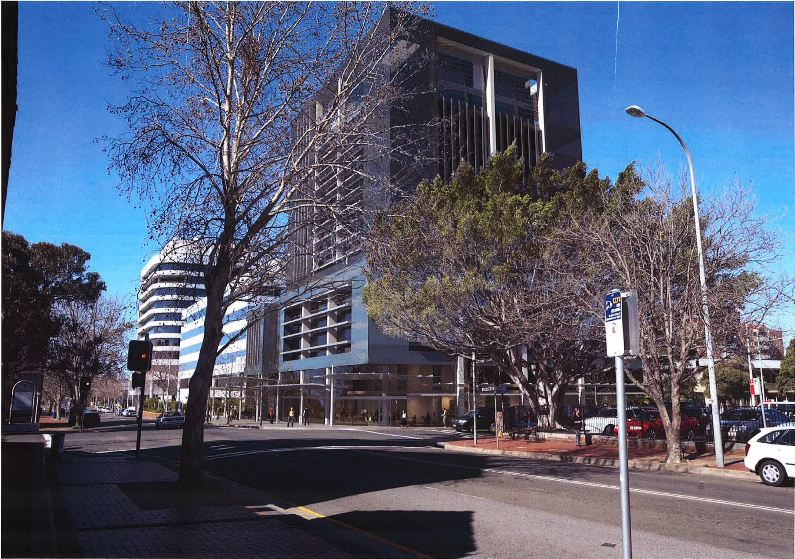
VIEW FROM WEST
