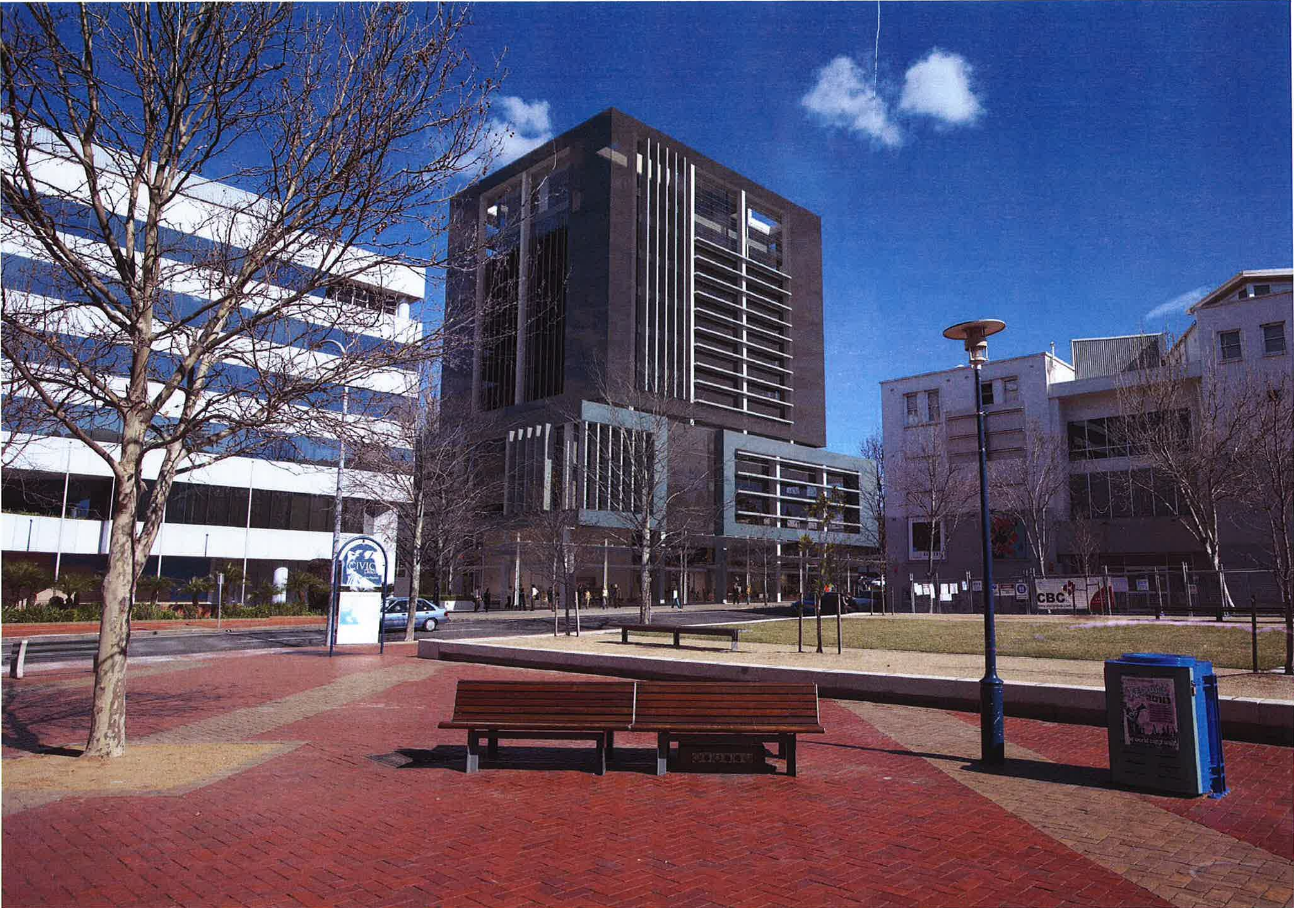
VIEW FROM NORTH EAST
